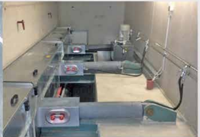
Robust hydraulic cylinder for walking floor movement
